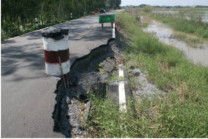
Figure 5: Slope failure of embankment.
