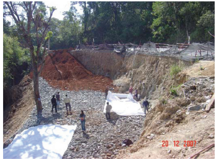
Figure 8: Drainage layer construction.
