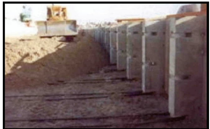
Figure 8: Back of Double-T Panels: Metallic strips connected to concrete buttresses (part of the concrete panels), and placement of 660 mm thick layer lift.
