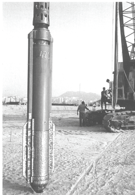
b) Vibroprobe at West Kowloon Reclamation.
