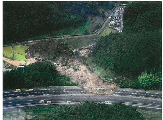
Figure 1: Embankment collapse in Yamaguchi by heavy rainfall due to Typhoon No.14 in 2005.
