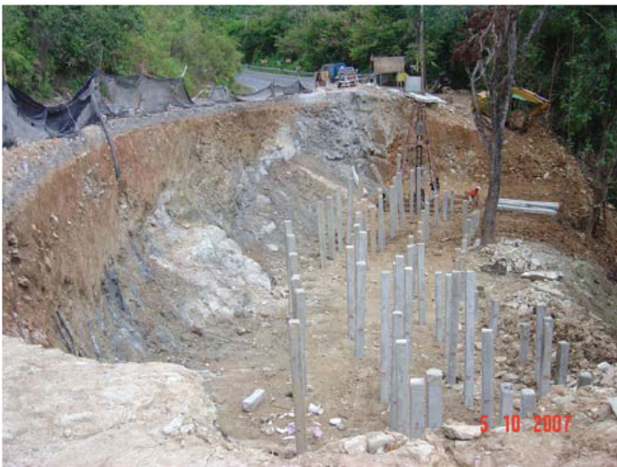
Figure 6: Piles construction.
