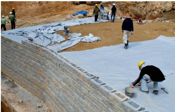
Figure 4: Installation of the composite reinforcing geotextile.
