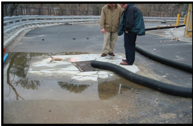
Figure 2: Concrete around surface water collectors to "repair" depression.
