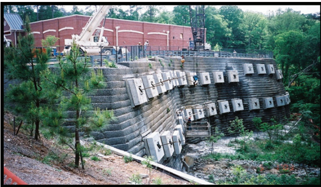
Figure 3: Anchors remedying the problem.
