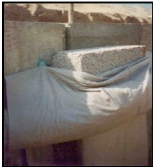
Figure 6: Facing Panels: Joints protected by no-fines blocks and nonwoven geotextile.
