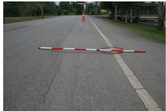
Figure 3: High settlement damage type.
