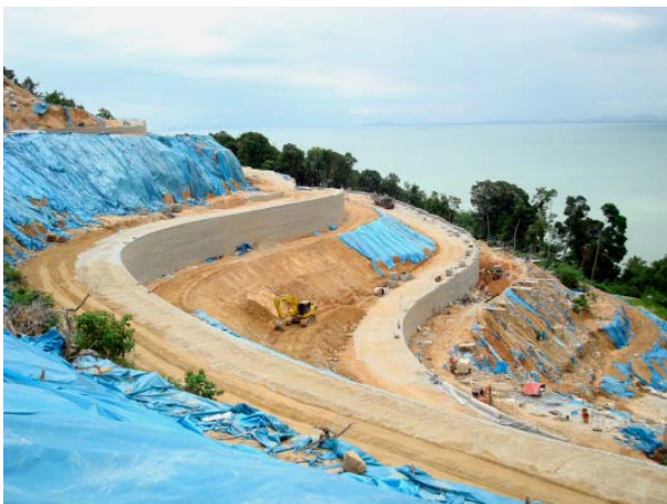
Figure 5: Construction of the reinforced soil segmental wall in progress.
