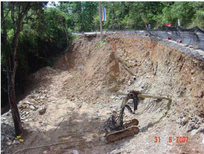
Figure 5: Soil nail construction.
