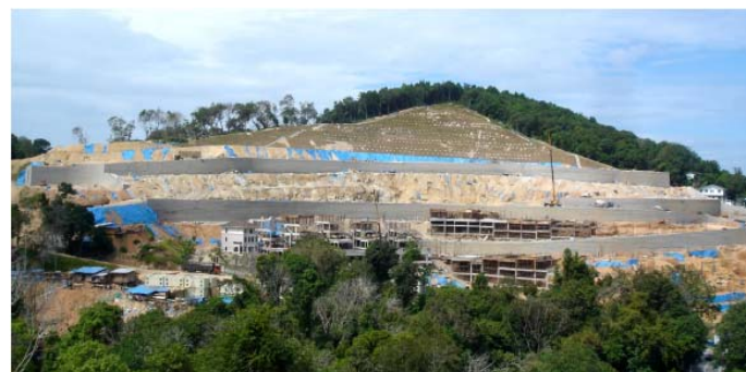
Figure 6: Overview of completed reinforced segmental retaining wall.
