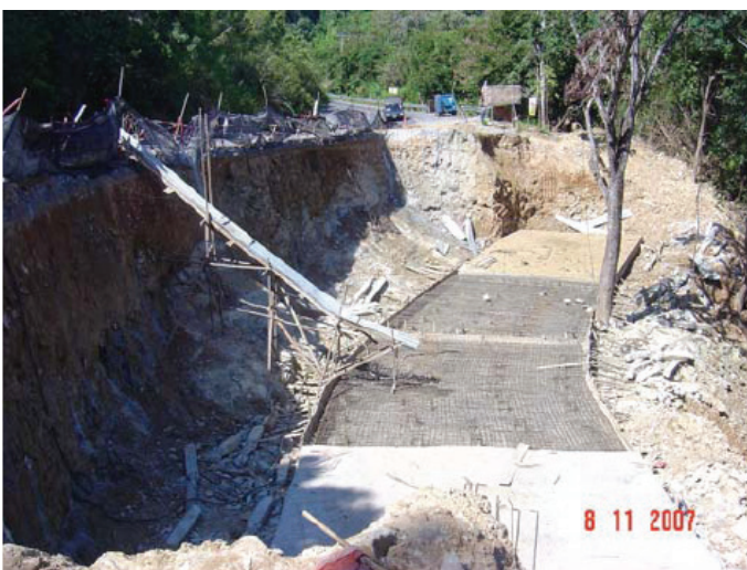
Figure 7: Footing construction.
