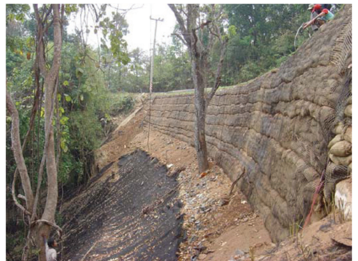
Figure 9: Geogrid (Miragrid®GX) reinforced slope and Erosion control mat (Polyfelt®Polymat) construction.
