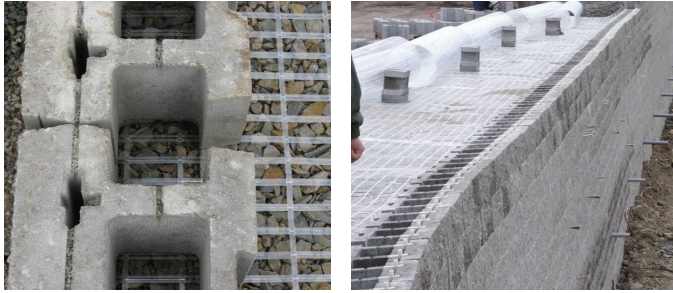
Figure 5: Block wall with friction connection under construction, Zanovica (SK), 2009.
