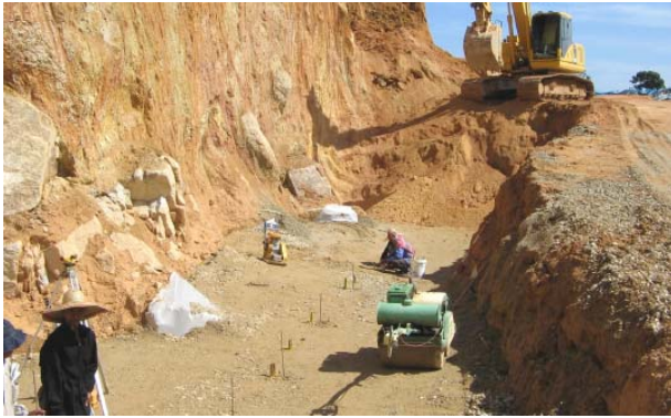
Figure 3: Ground replacement with well compacted granular fill and reinforced with composite reinforcing geotextile.
